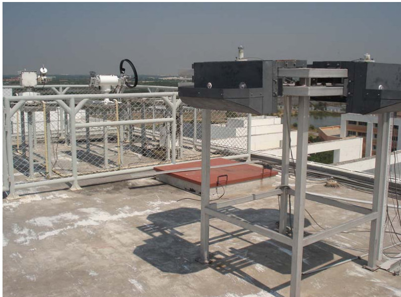
Daylight measurement station
